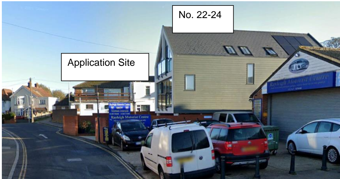
Photo 1: Street scene photo of Bellingham Lane which shows No. 22-24 and the application site.
