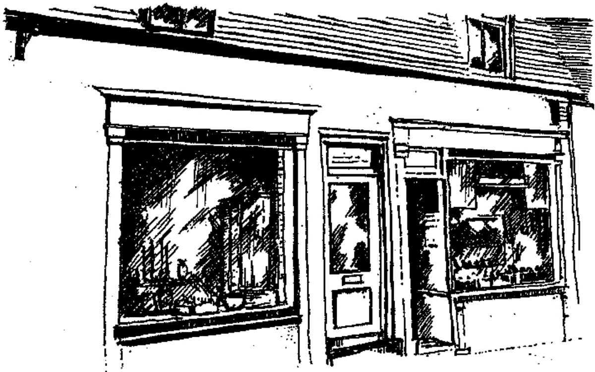
Attractive shop fronts with pilasters and fascia, marred by the insertion of plate glass windows
