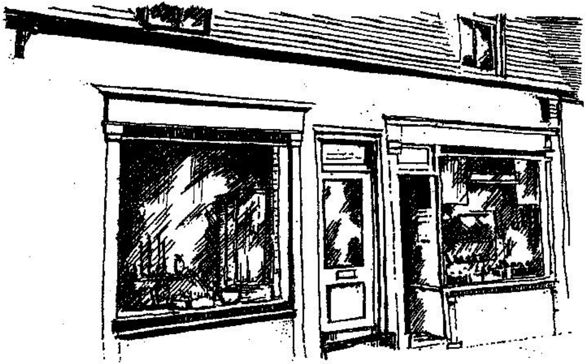
Attractive shop fronts with pilasters and fascia, marred by the insertion of plate glass windows
