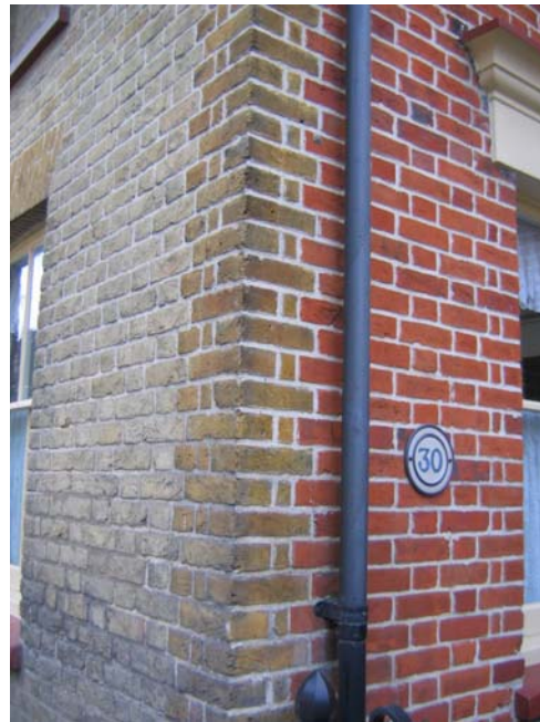
Fig. 11 Angle of nos 30-32 South Street. White bricks were used for the façade, with stocks for quoins and window lintels, and red bricks in the side.
