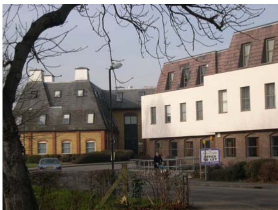
Fig. 31 Locks Hill, Cottis House and Canewdon House.
