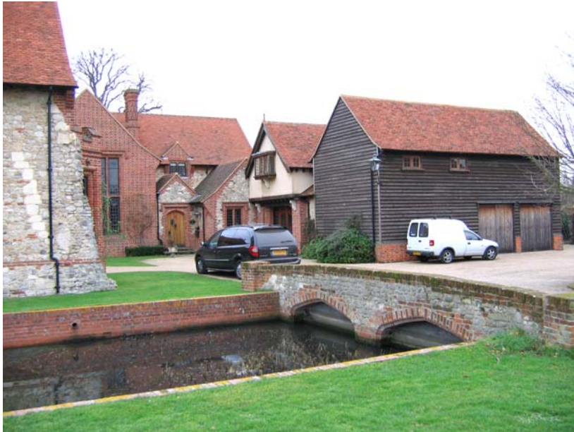
Fig. 17 Rochford Hall, a view of the residential conversion of the former barns area.
