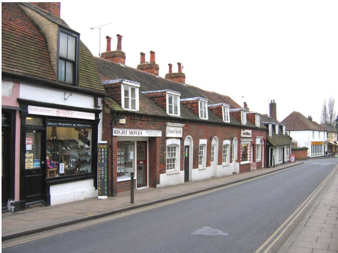
Fig. 45 West Street, cottages at west end (nos 53-69).
