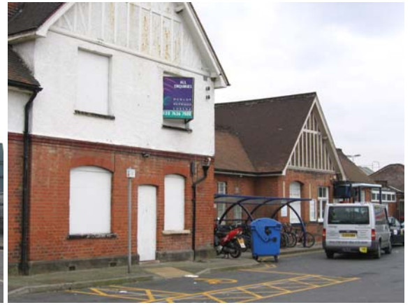
Fig. 38 Rochford Station, boarded up former station master's house.
