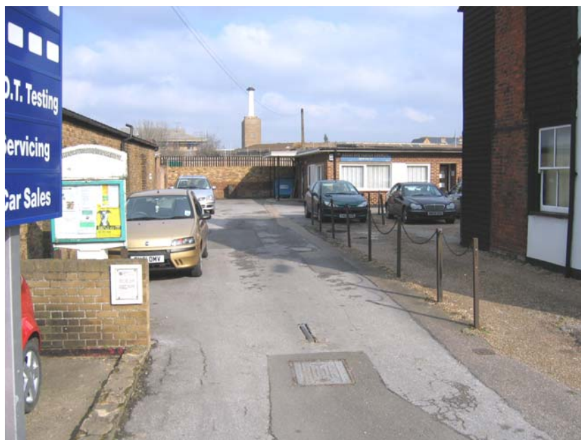
Fig. 35 West Street, depressing view between Whittingham's garage and Sovereign House to the parish council offices. In the background, the former hospital boiler house.
