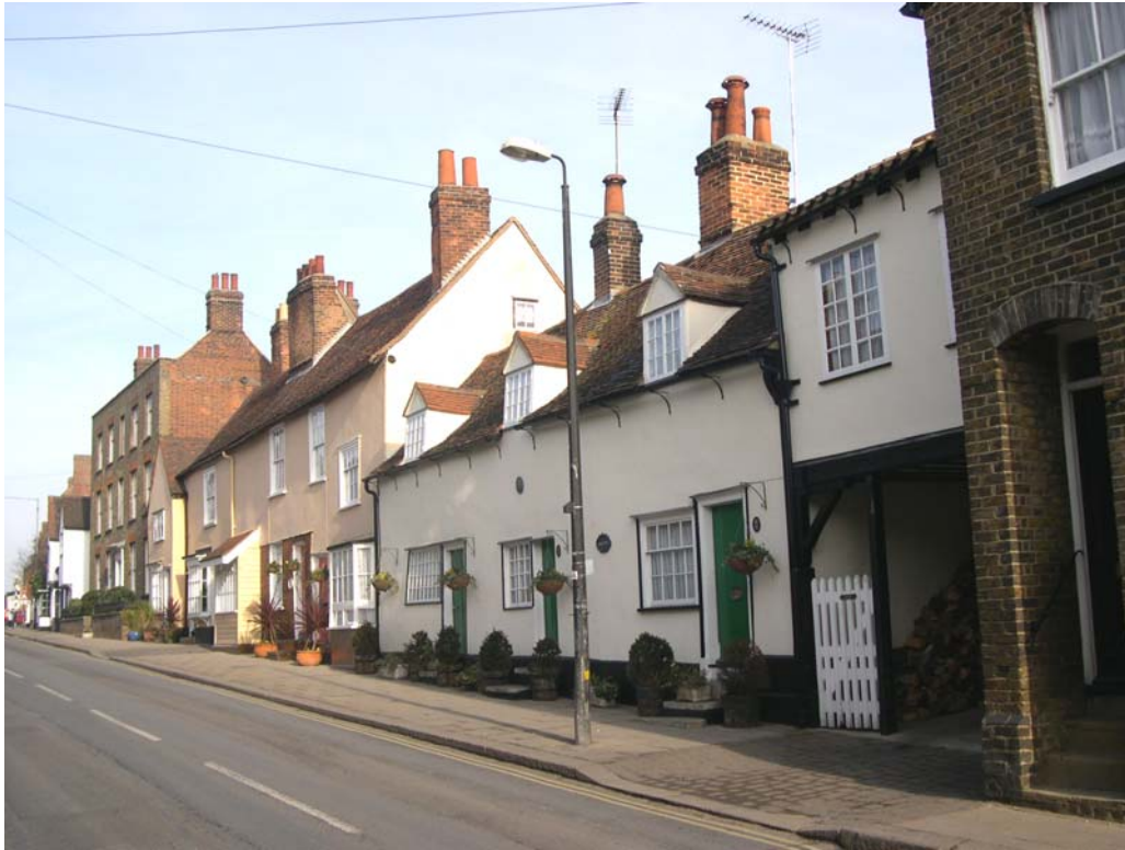
Fig. 23 South Street, east side, nos 19-35.
