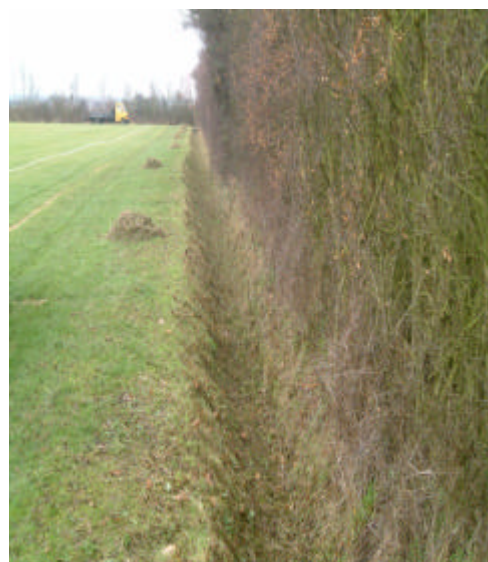
Clearing the ditches
