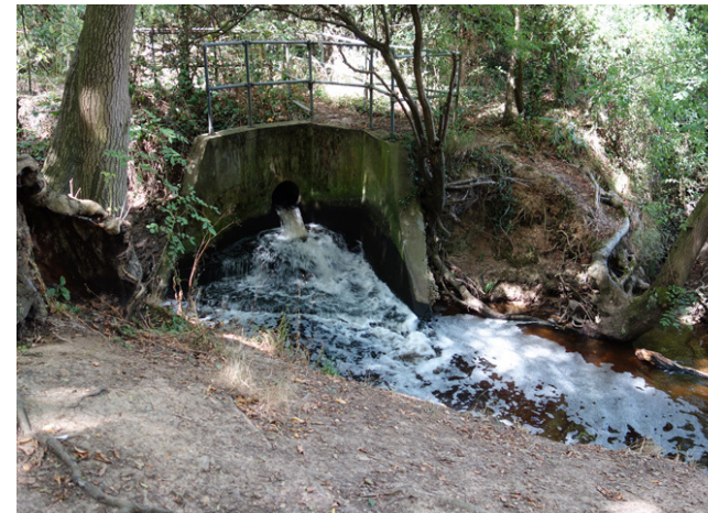
23 Drainage connections discharge into the River Roach
