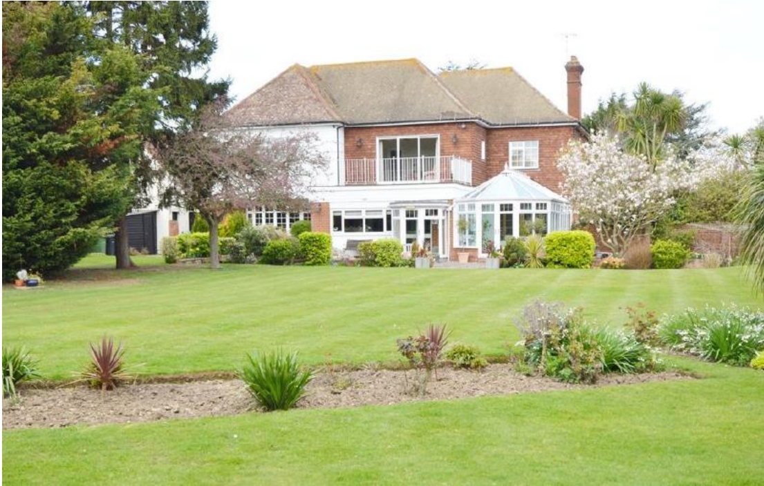
Photo: Previously existing rear elevation dwelling prior to demolition
