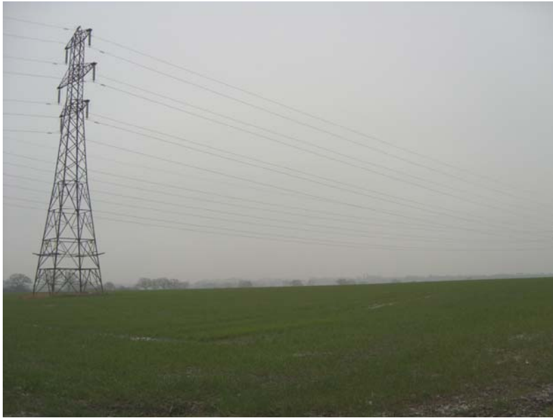
Viewpoint 1 (Looking north west)
