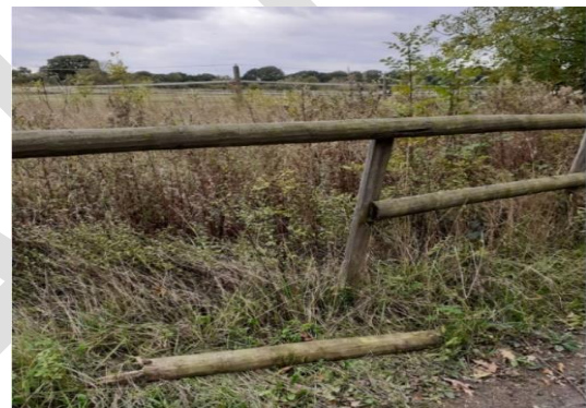
Figure 47: some areas need maintenance.
