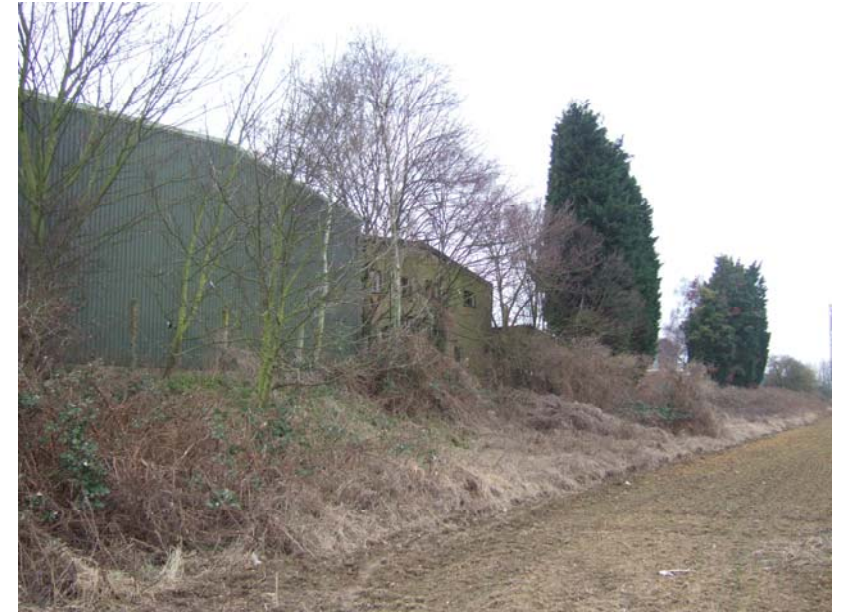
Viewpoint 5 (Looking south/south west)
