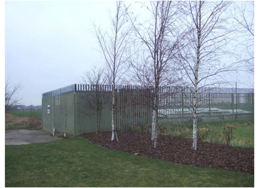
Viewpoint 3 (Looking north west)
